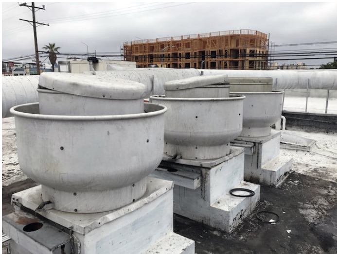
Three rooftop exhaust fans controlled by the DCKV system at Versailles.
