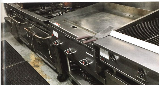
The DoubleTree cookline now features a griddle with thermostatic controls that help control energy consumption.
